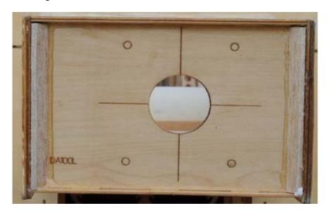
27. The distance from the front face of the motor box to the motor drive washer is <u>7.25 inches</u> (this is the length of the DA-120 with 1 inch standoffs, the DA-100 requires 3/4 inch standoffs). Drill holes at the marked locations and install the engine using the recommended mounting bolts.
