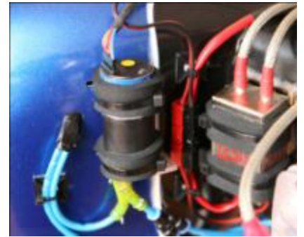
The ignition and the smoke pump mounted at the dome
